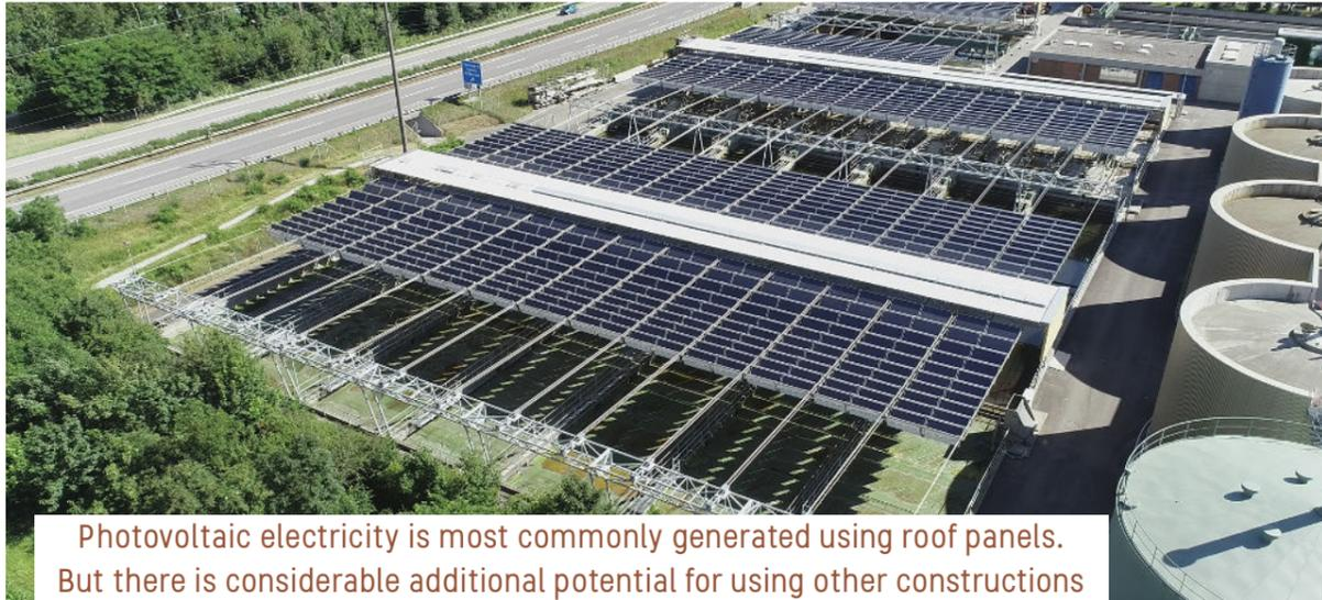
Photovoltaic electricity is most commonly generated using roof panels. But there is considerable additional potential for using other constructions that up to now has been seldom exploited. The solar fold-out roof from dhp technology (in Zizers, Canton of Graubünden) is deployed over treatment tanks in sewage plants to generate renewable energy.
