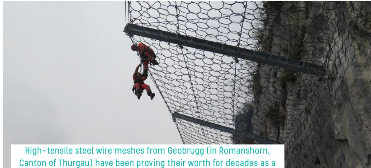
High-tensile steel wire meshes from Geobrugg (in Romanshorn, Canton of Thurgau) have been proving their worth for decades as a protective measure against rockfalls, landslides and other natural hazards. In future, the company's products could also help mitigate the effects of climate change.
